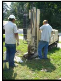
Installation of Monitoring Well
