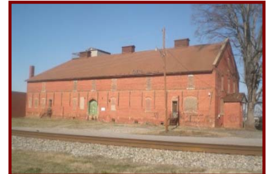
Former Piedmont Wagon – Southern Facade
