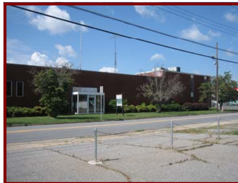
Former Regal Manufacturing – Northern Facade
