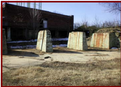
Former S&W Chemicals, Inc. – Northern Facade
