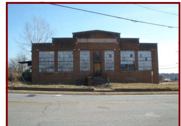
Former Holler Hosiery Mill — 883 Highland Avenue Southeast
