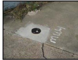
Completed monitoring well at the SOC Station.
