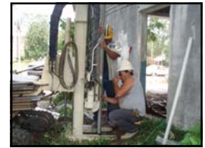
Installation of a monitoring well at the SOC Station.
