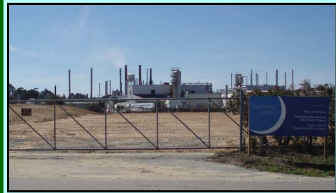
SDS Property after demolition through the CDBG Grant funding
